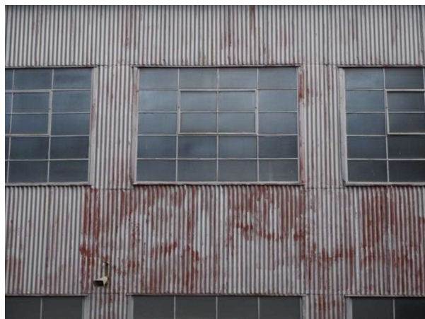
Building Three, standard window unit (four by five) with central pivoting window
