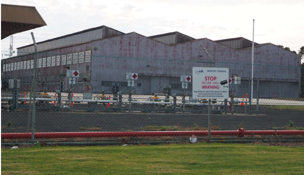
Building Three – south-east part from Drake Street, note extended clerestory windows with muntins/vertical glazing bars
