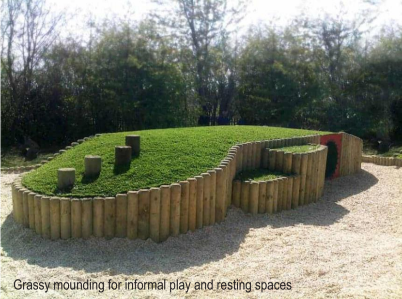
Feature stepping log wall retaining wall
