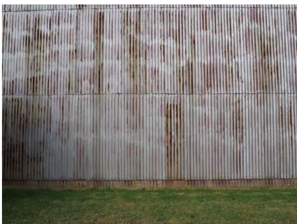
Building Three, close-up of east elevation cladding, note concrete slab/plinth and prominent header nails
